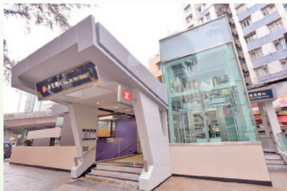
接駁路面及港鐵車站大堂的升降機 External lift connecting street level to concourse
