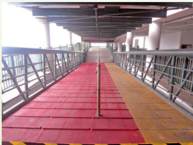
鋪有防滑物料及設有槽紋的碼頭斜道 Ramps with anti-skid gangplanks and grooves at pier
